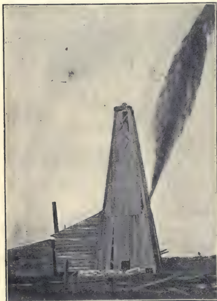
FIG. 105—Torpedoing an Oil Well near Petrolea, Ont.
